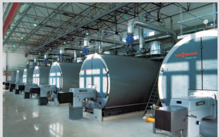
Xi'an, central China: The seven WKG gas burners in this heating centre provide more than 50000 residents in the Zi Wei garden district with 115 MW of heat
