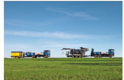
Borehole drilling by BauGrund Süd
