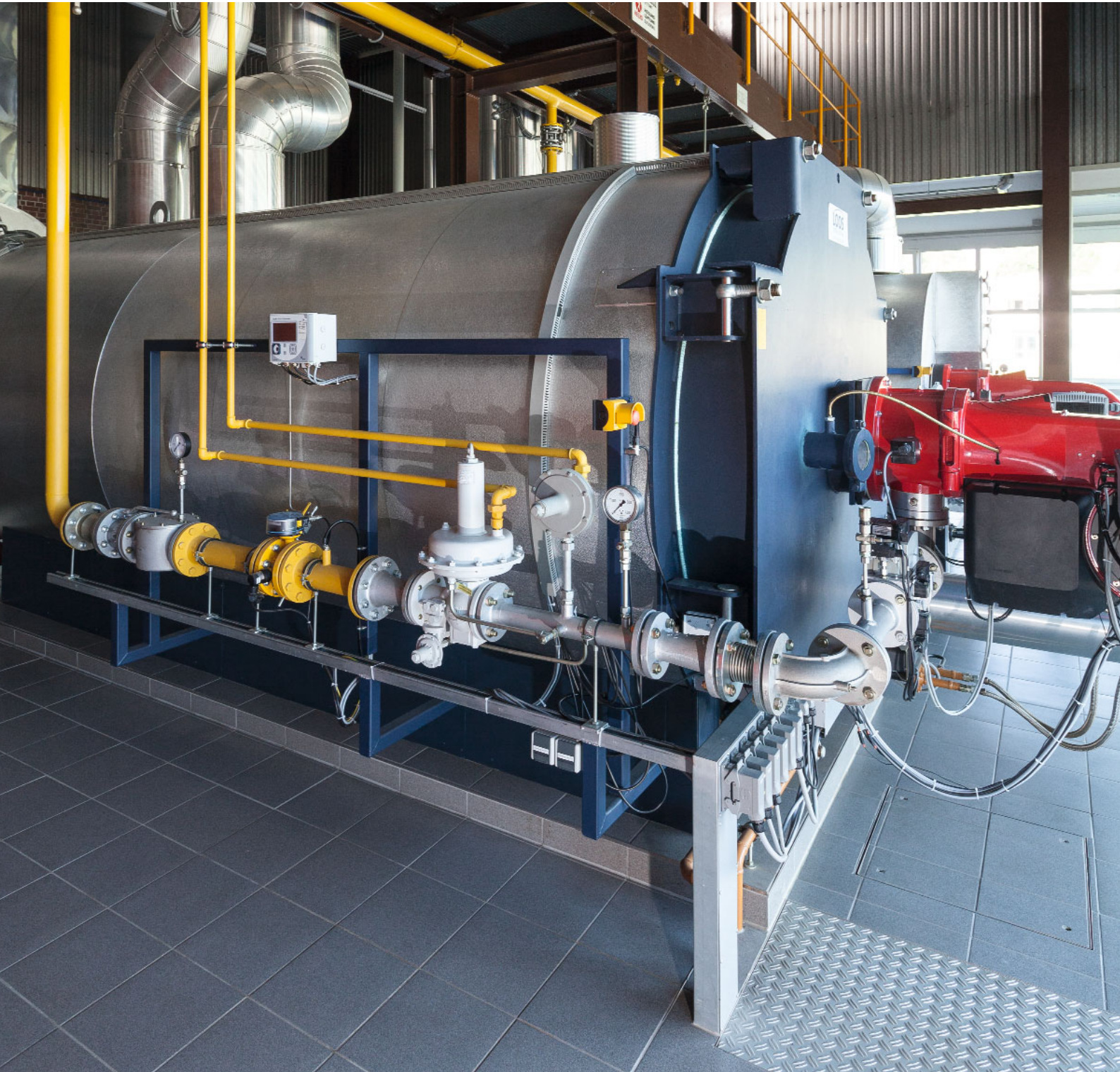
High-pressure gas supply – Heating centre at Weishaupt's main works in Schwendi, Germany
